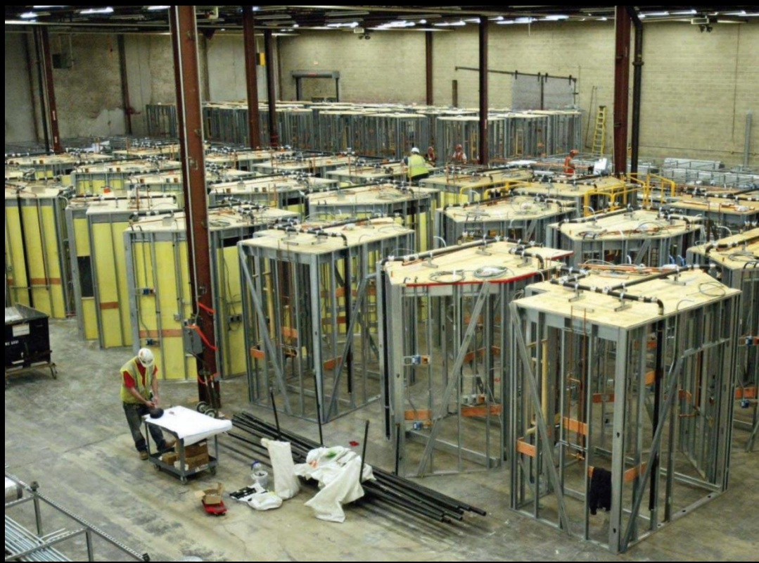
Prefabricated Bathroom Pods at Miami Valley Hospital
